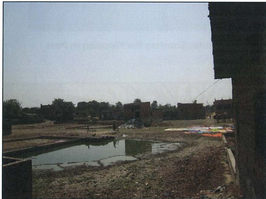
Photo: Showing lack of Internal Drainage System
