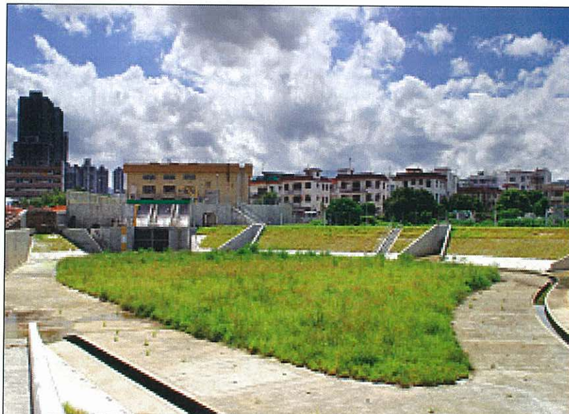
Village Flood Pumping Scheme in Ma Tin Tsuen, Hong Kong
