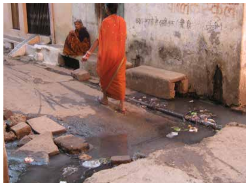
Open drainage in Nariyal Kheda, Bhopal
