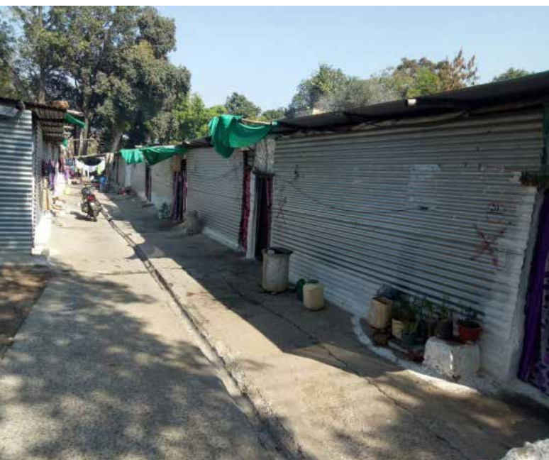
Tin shed houses in Bhadbhada Basti and Jawahar Nagar, Bhopal
