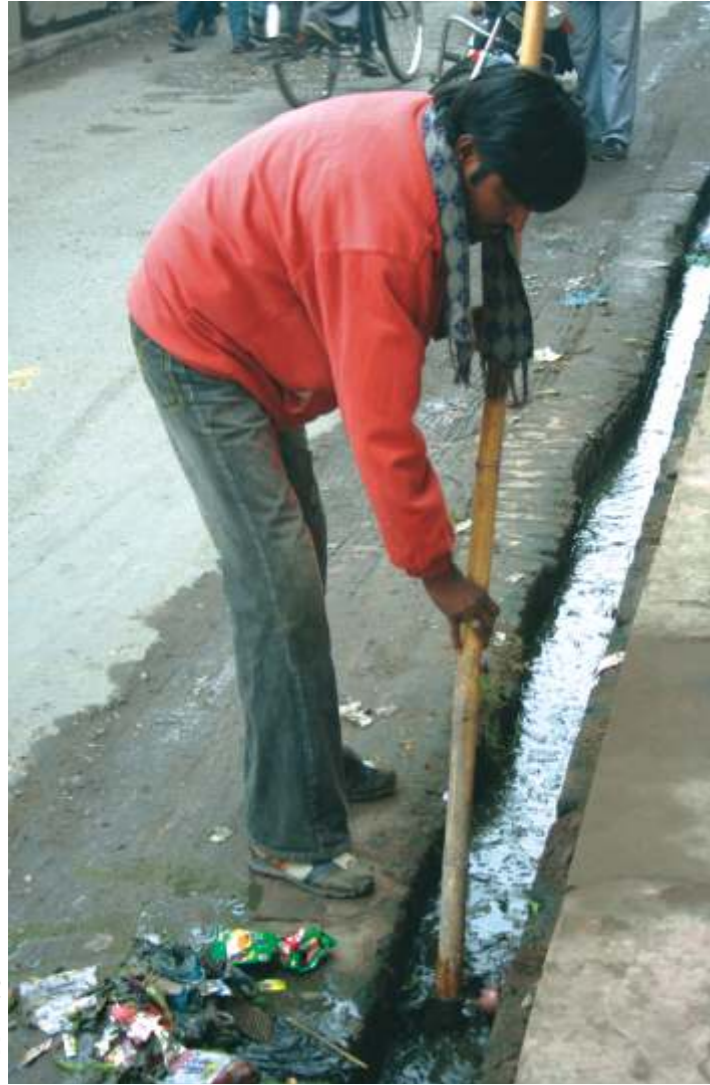
Photo 5 | Cleaning up drains
