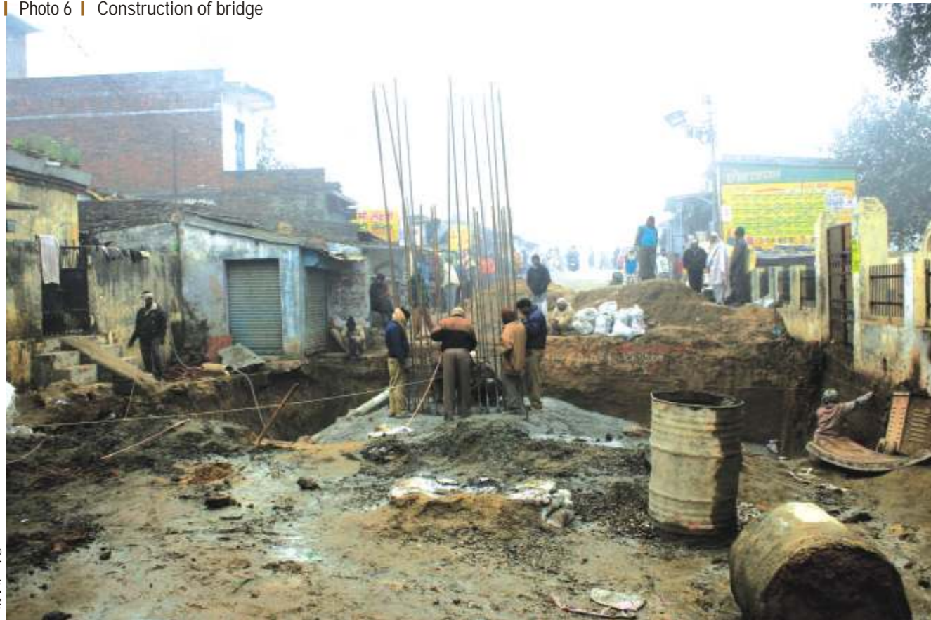
Photo 6 | Construction of bridge
